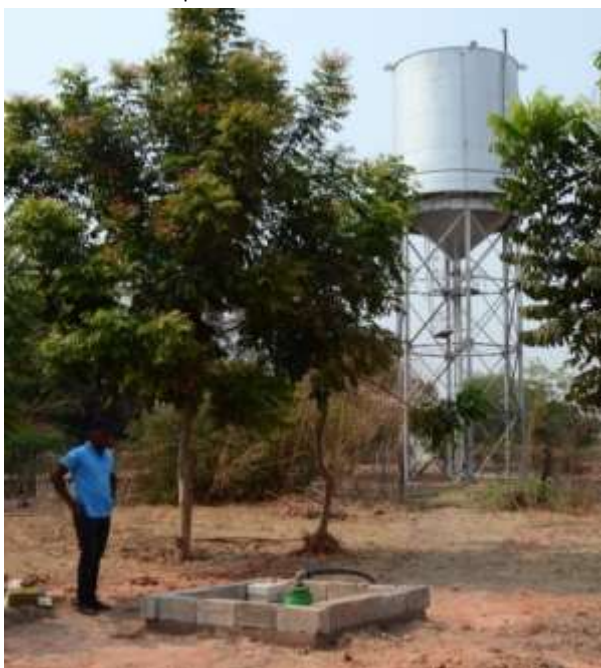
Before the water pipe is connected to the tank, the water runs outside until it is clear. For safety reasons, four solar lamps were mounted on the tower.
