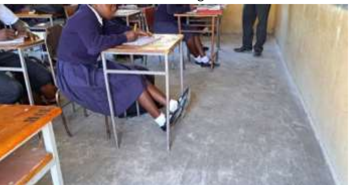
Top: After the cement floors have been stripped, they are soaked for a few days to harden the cement. Below: The floors are back to their former glory and the school furniture is stable again.
