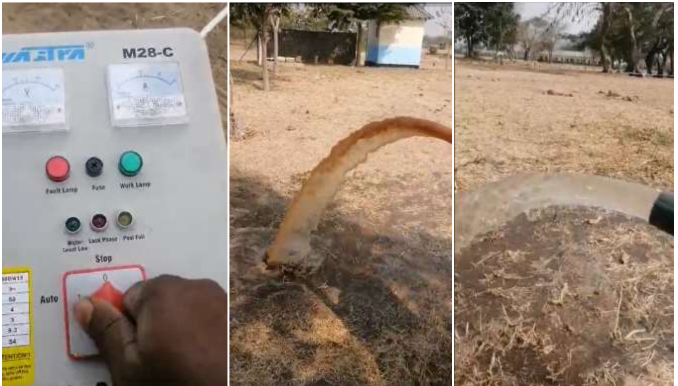
Before the water pipe is connected to the tank, the water runs outside until it is clear. For safety reasons, four solar lamps were mounted on the tower.
