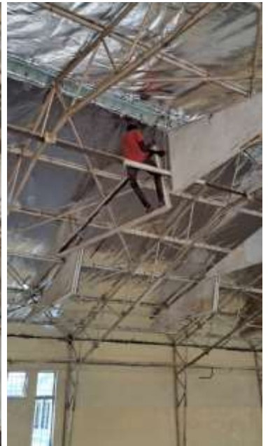
An aluminium foil was attached underneath the corrugated metal roof as thermal insulation. In addition, the foil brightens up the building by reflecting the light. The insulation effect of the foil is remarkable.
