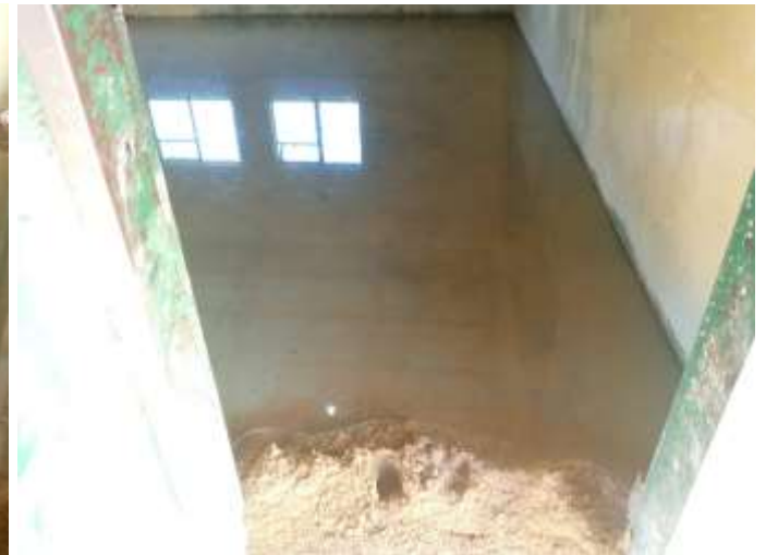
Top: After the cement floors have been stripped, they are soaked for a few days to harden the cement. Below: The floors are back to their former glory and the school furniture is stable again.
