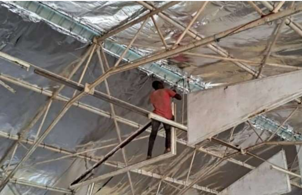
An aluminium foil was attached underneath the corrugated metal roof as thermal insulation. In addition, the foil brightens up the building by reflecting the light. The insulation effect of the foil is remarkable.
