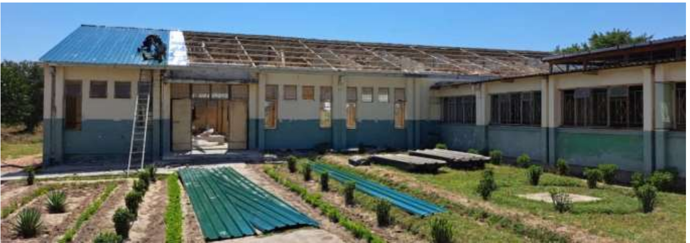
An aluminium foil was attached underneath the corrugated metal roof as thermal insulation. In addition, the foil brightens up the building by reflecting the light. The insulation effect of the foil is remarkable.
