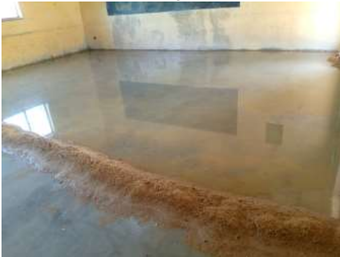
Top: After the cement floors have been stripped, they are soaked for a few days to harden the cement. Below: The floors are back to their former glory and the school furniture is stable again.
